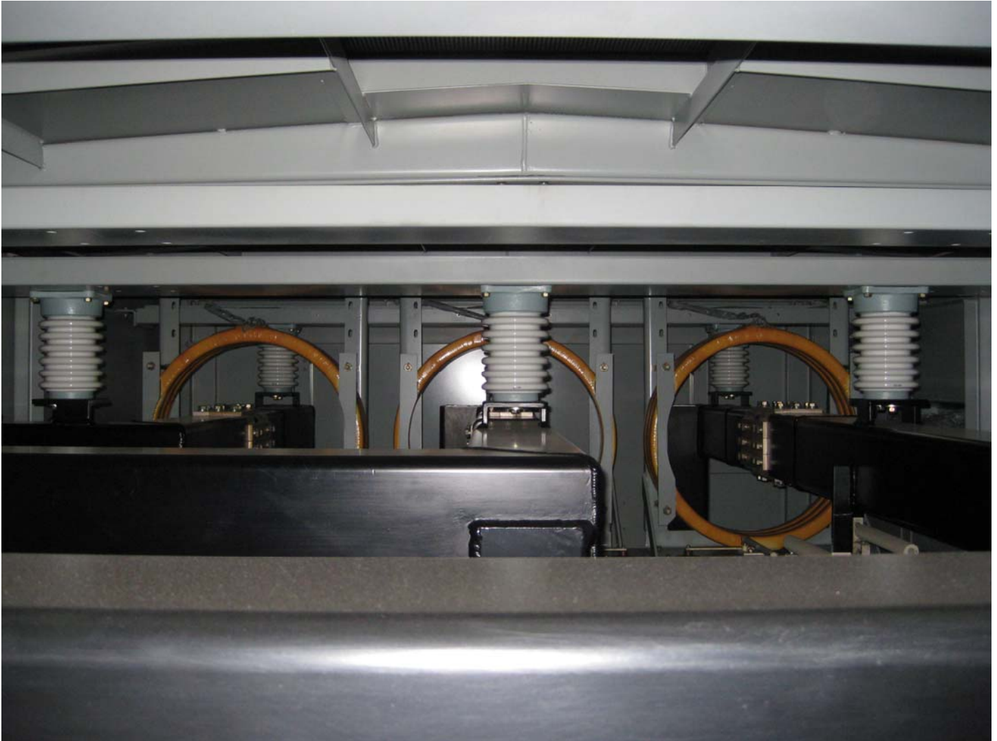
Terminal Ends of Windings with Terminal CTs
